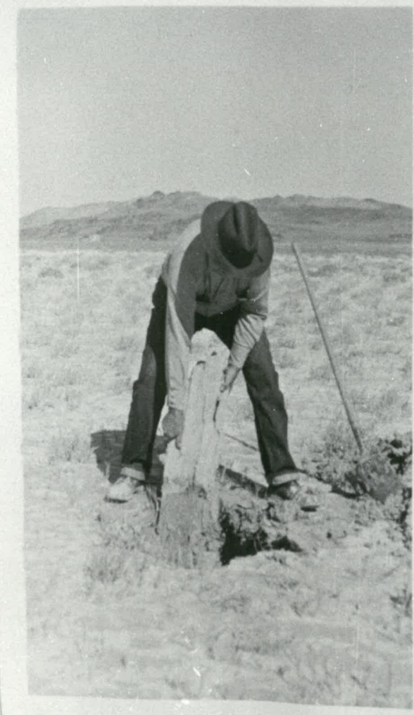
Either 1955 or 56 58 Ward McCarty digging up an old telegraph pole stump 8-8 inches at butt. 165 feet apart--10 rods- 32 to the mile. One half mile west from Boyds
